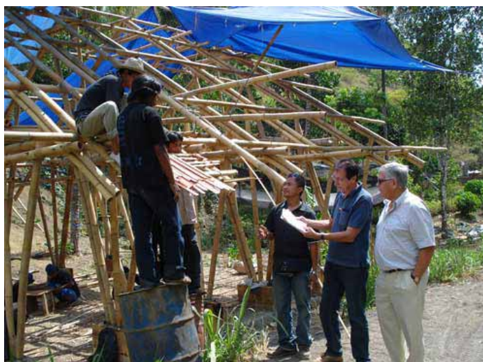
Constructing the model bamboo house
