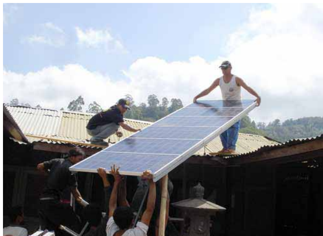
The solar cell is being intalled at EBPP Bunga school
