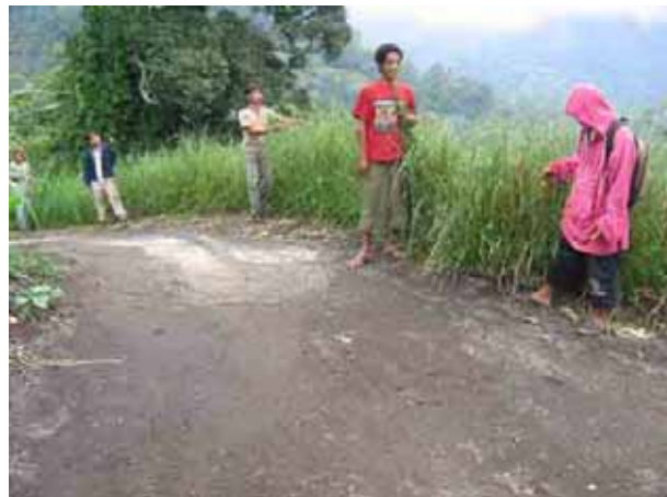
Vetiver hedges protect step concrete stabilized road to Cegi
